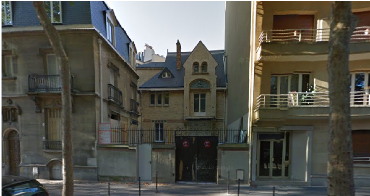
Rue Molitor, Paris
